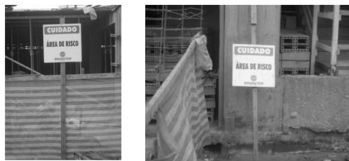
Figure 5: The Mobile Signs
